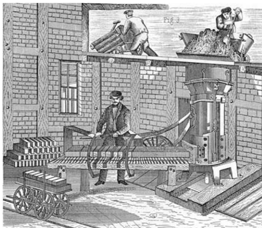
Fig. 16 First upright auger extruder powered by steam, 1858
